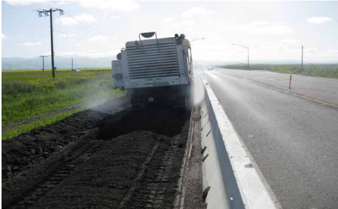
Grinding of the widening at Shore Rd.
