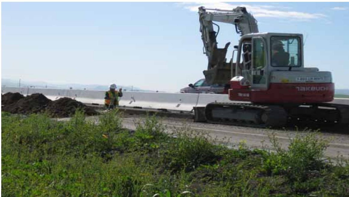
Pavex digging Stage 2 Traveled way
