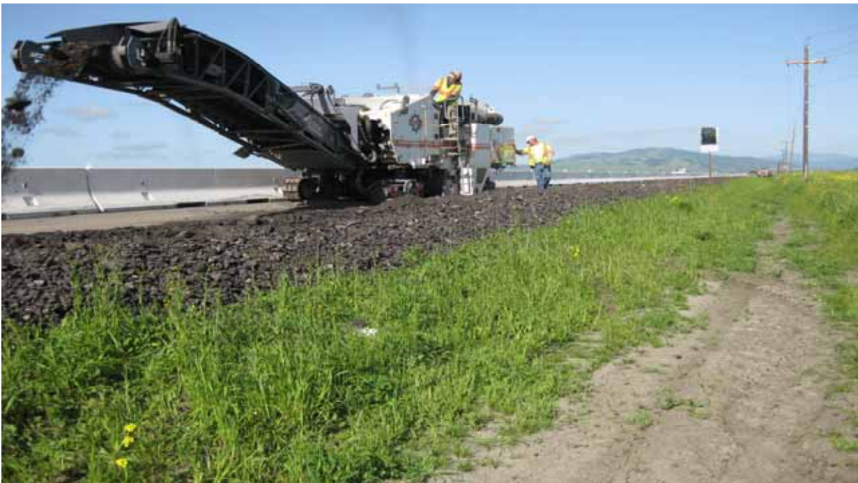
• Grinding @ Shore Rd
